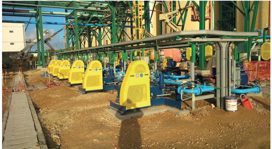
*HPT triplex plunger pumps from ABEL are being used for gland seal water supply*
